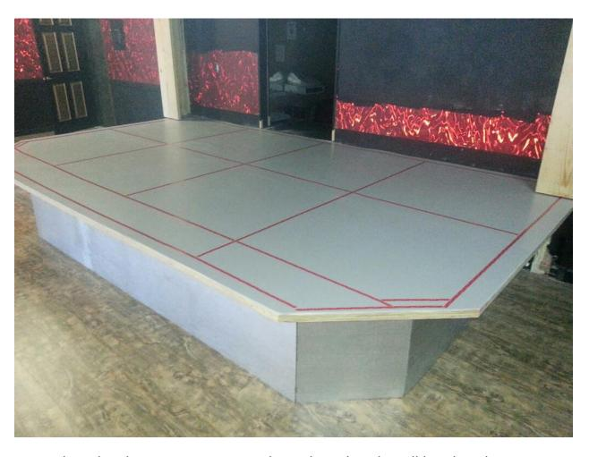
Step three lay down 3M VHB tape where the gel packs will be placed. See more photos below.
